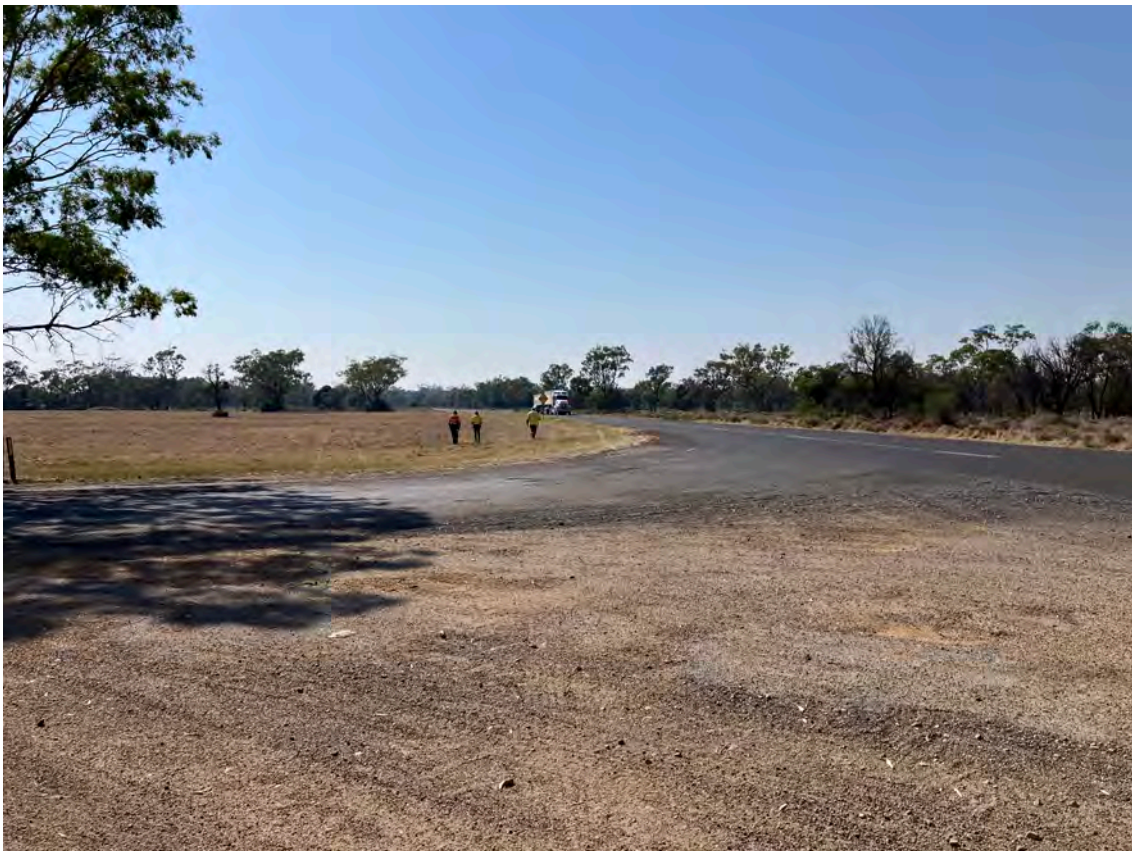
Figure 8. Work area for the upgraded site entrance off the Gwydir Highway.
