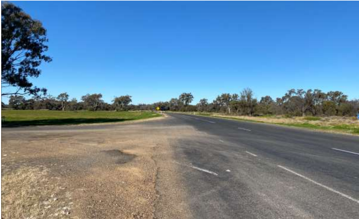
Figure 29: Sight Distance – View east along the Gwydir Highway from existing site access. Sight distance of over 500 metres.
