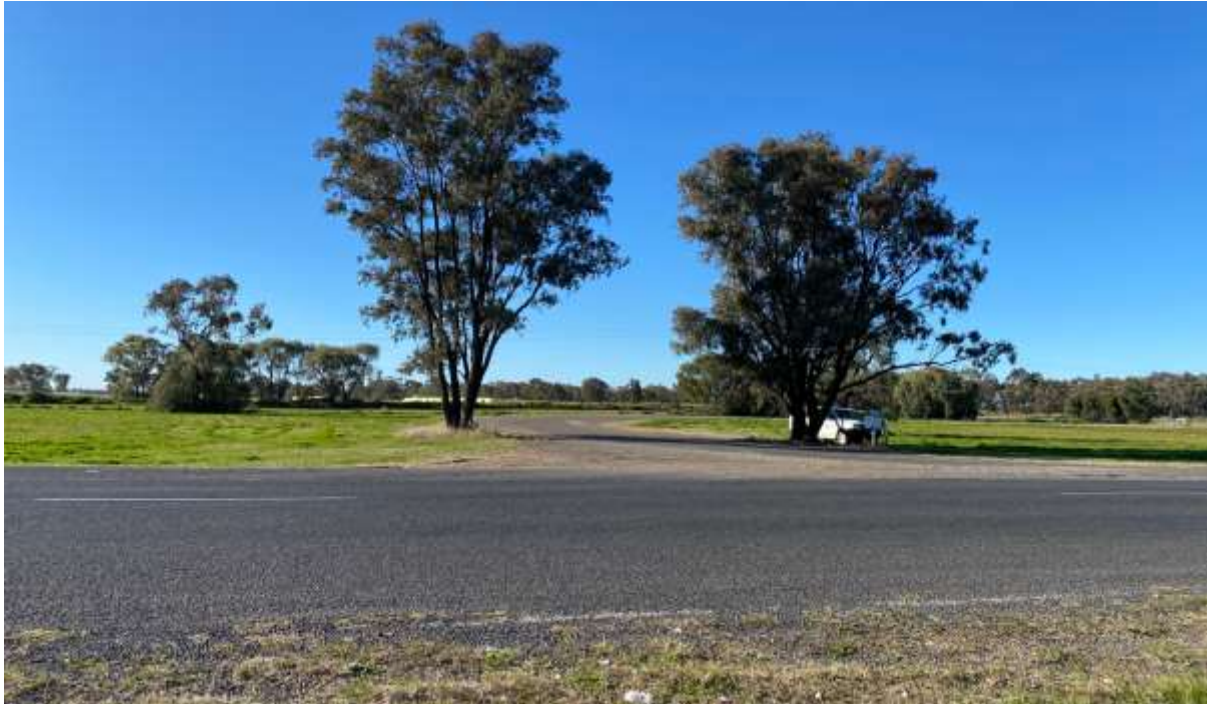
Figure 27: Existing property access from the Gwydir Highway
